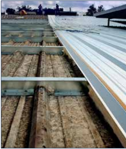
Retrofit framing over an existing roof
