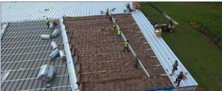
Workers creating airspace between the old and new roof
