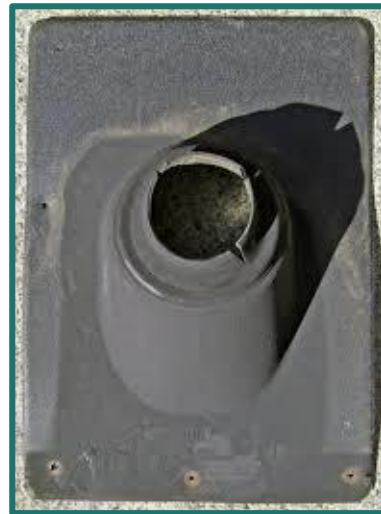
Recycled rubber degrades due to UV exposure.
