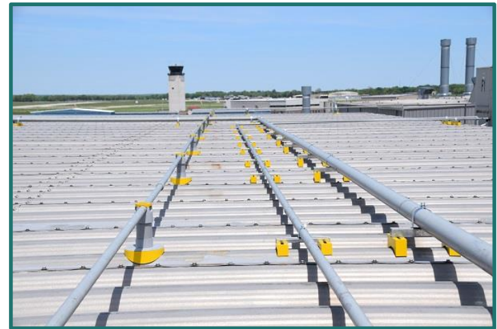
AFTER the installation
