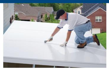
Peel & Seal PowerBond<sup>®</sup> White 250 utilizes the same benefits of Peel & Seal<sup>®</sup>, but is designed specifically to tape seams on insulated aluminum panels.
