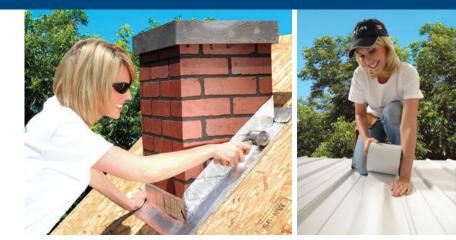
Peel & Seal® is an ideal choice as a flashing material around chimneys, roof vents, stack pipes and other difficult to waterproof items. Peel & Seal® can also be used to completely cover, flash seams or repair metal roofing systems.
