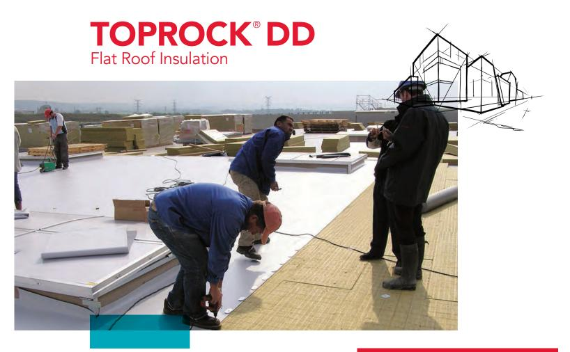
ROCKWOOL TOPROCK® DD is a high-density, uncoated stone wool insulation board for low-slope roof applications. TOPROCK® DD is a suitable substrate board for all low-slope roof decks and is compatible as the substrate for mechanically attached membrane systems.
