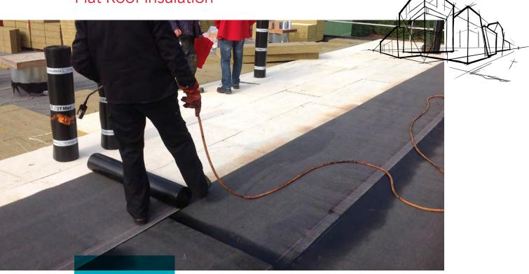
ROCKWOOL MULTIFIX<sup>™</sup> is the first stone wool insulation product with a mineral-coated fiberglass facer that is compatible with multiple attachment methods including torched, hot-mopped, self-adhered, cold-adhered and liquid systems.
