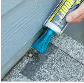
Over roof nails
