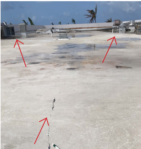
Mechanical equipment that became airborne on the CEP building during the hurricane caused skid marks in RoofPROmembrane.
