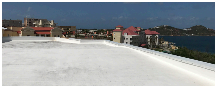
Sikalastic® RoofPRO membrane on the medical building roof at the American University of the Caribbean in St. Martin.
