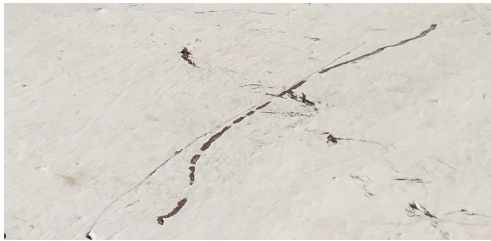
A closer look at skid marks in RoofPRO membrane.
