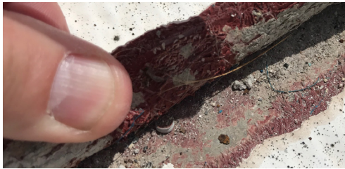
Bonded membrane does not allow water to migrate laterally
