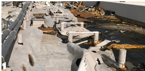
Torn off loose laid membrane system.
