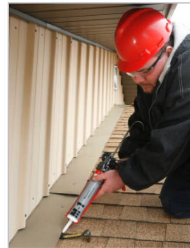
M-1 water block underneath metal flashing
