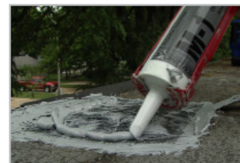
Patching a leak as part of a 3-course flashing repair
