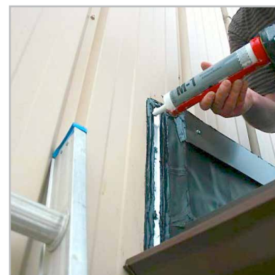
Sealing termination bars
