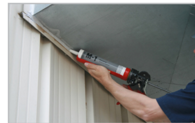
Sealing HVAC flanges
